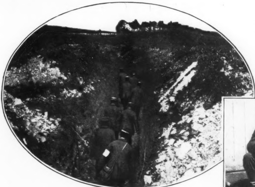
THROUGH THE COMMUNICATION TRENCH
